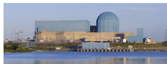
Exelon's Clinton nuclear plant.
